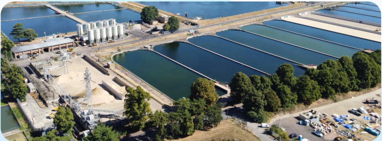
Filter beds at Hampton Water Treatment Works
