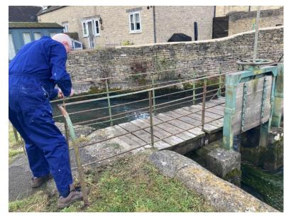
Preparation involved wire brushing and sanding the iron railings and sluice gate frames to remove the rust and loose paint.
