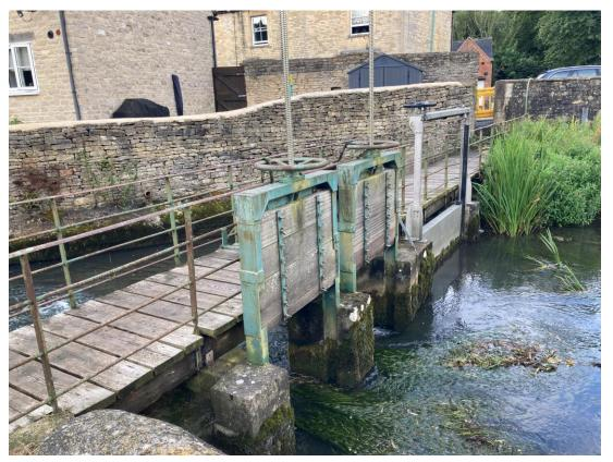
There are three sluice gates at the weir, plus a pedestrian bridge with iron railings.
